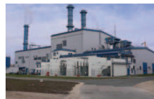
Left: Siemens 45MW SGT-800 gas turbine may be used independently for power generation or, as above, in CHP mode
